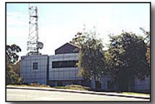
Figure 2-19 Fire Communications Center
